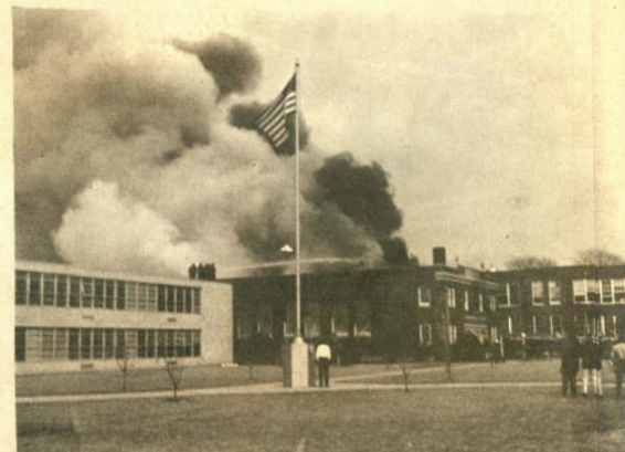
LOOKING EAST smoke may be seen rising from old section of Bellport Junior-Senior High school. United States flag waves in front of new wing to left. Firemen direct water in gymnasium, center. The $500,000 fire destroyed the old section.
